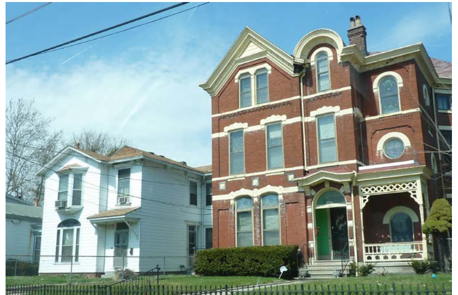
A brick Italianate next door to a simple Victorian
