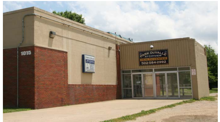
The current Park Duvalle Health Center at Cityview Park
