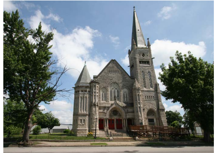
St. Peter's United Church of Christ is on the National Register of Historic Places and is located across the street from Beecher Terrace
