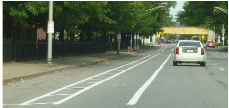
A bike lane was added to Muhammad Ali Blvd in spring 2015.
