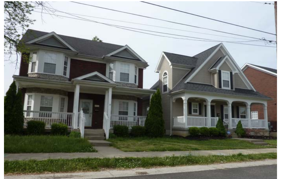
Recent housing construction in Russell
